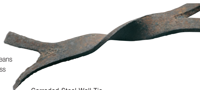
Corroded Steel Wall Tie
