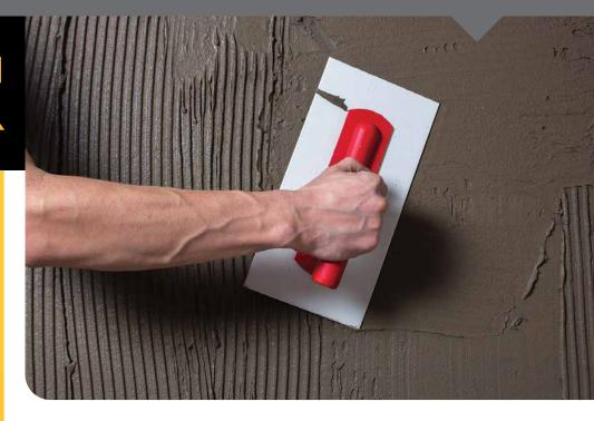
Wykamol **Renovation Plaster** is designed to have similar properties to a 1:1:6 cement:lime:sand plastering mortar. Lightweight, perlite aggregates replace a portion of the sand to reduce heat loss and condensation.
