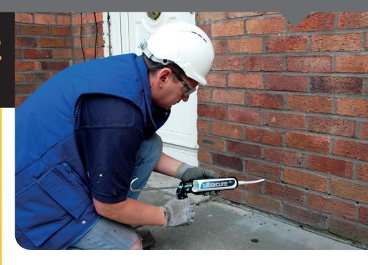
The cream is delivered by hand pressure from the appropriately sized applicator gun into a series of holes drilled into the mortar course.
